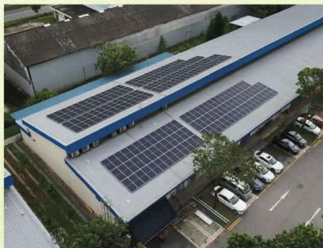
Implementation & Installation of PLC's Solar Panels
