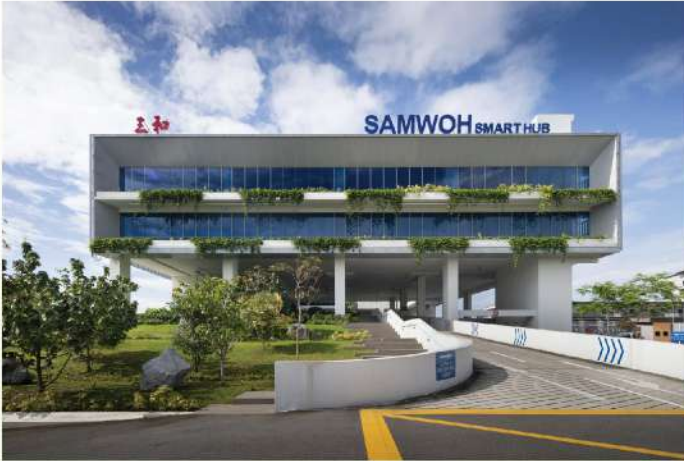
SamWoh Smart Hub Building
